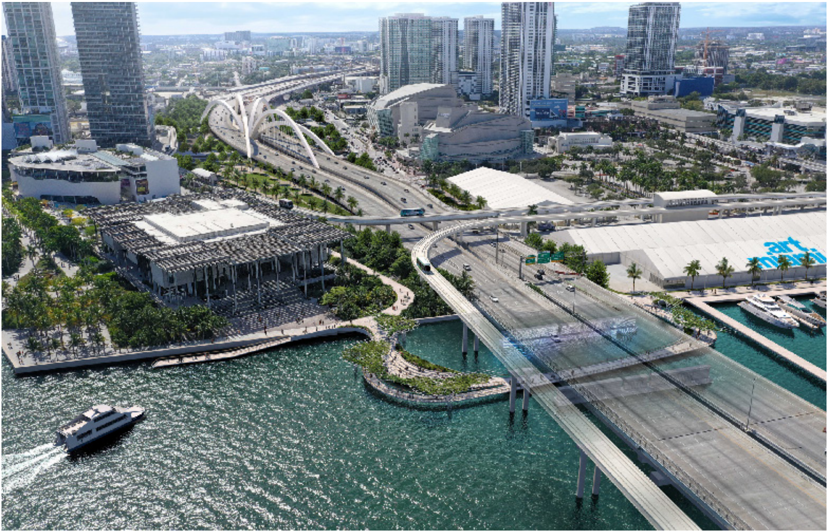
Miami DDA Pedestrian Bridge
